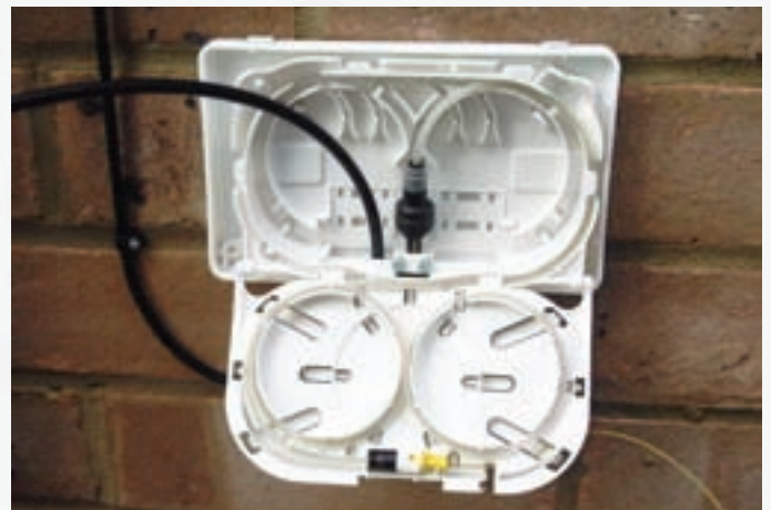
Typical use of a John Guest Gas Block/Fibre Lock & Straight Reducing Connector in a customer splicing point enclosure.
