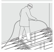
Remove any loose debris, and ensure all pipes are securely fitted to provide a flat and stable surface for the flooring.
